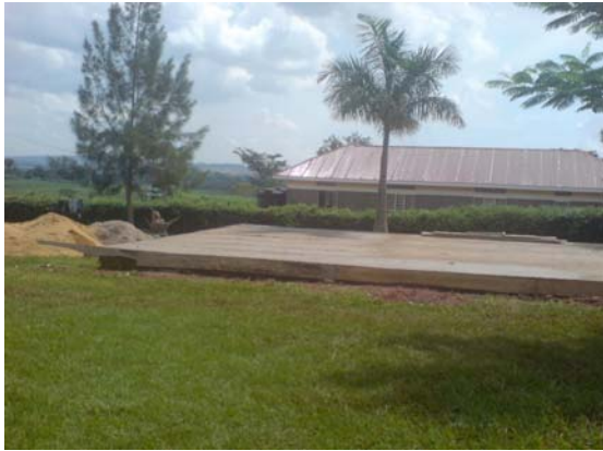
Construction of the Labour and Maternity ward under construction above
